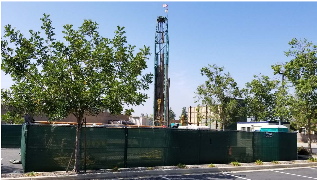
Grand Avenue Well Drilling Activities
